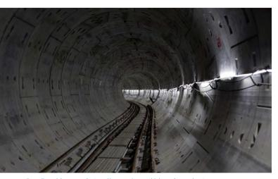
Deep Tunnel Sewerage System, Singapore's superhighway for used water PHOTO CREDIT: PUB
